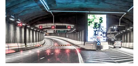
When driving through the tunnel of the Norra Länken motorway in Stockholm, you may be amazed to see a fully graphic artwork with changing colours. The fully graphic installation of moving images boasts 16 million colours with a 16 mm pixel pitch on an area measuring approx. 4,500 mm × 6,100 mm, as well as featuring 288,768 LEDs with a power consumption of just 700 W.
