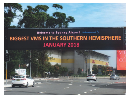
Top Image: VMS used to display live parking availability and parking guidance Bottom Image: The largest VMS in the Southern Hemisphere used for lane control at Sydney Airport
