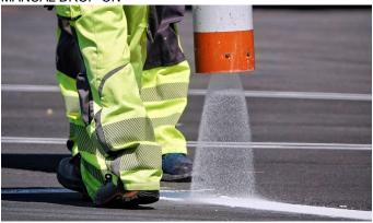
In addition to drop-on applications, SWARCOFLEX retroreflective glass beads can also be integrated directly into the road marking matrix during the production of thermoplastics, cold plastics, or similar marking materials. These products are ideal for use in various environments, including highways, urban roads, parking lots, and airport runways.
