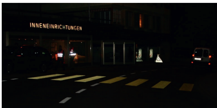
Figure 6. Yellow pedestrian crossing in Switzerland; “zebra” stripes on the left reflectorized with GB characterized by RI 1.6–1.7 (“Premium”) and on the right with RI 1.5 (“Standard”).
