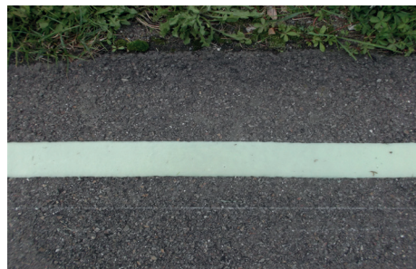
2-component afterglow plastic as edge line
